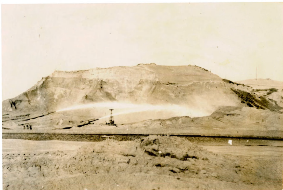
Pl. 6.- Cut being made at Hyperion which shows active dune sands above consolidated ridge.
